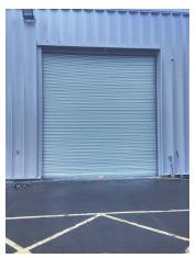
A safeguard 76 Electric operated roller shutter door 3800mm (W) x 5000mm (H) with wind anchored guide system was also installed in place of an existing worn and damaged shutter.
