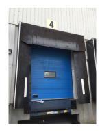
Our work involved refurbishment of another 22no existing loading bays. Each loading bay door was completely stripped of the damaged/worn panels and replaced with new door panels. External silver finish and with a row of vision panels.
