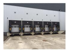
The existing dock shelters were too badly worn and damaged to refurbish. A&C dismantled the existing shelters and replaced with 22no new dock shelters, 22no new pairs of dock buffers and 22no new traffic light systems.
