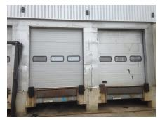
Phase 1 involved the refurbishment of 22no loading bays. The existing loading bay doors were completely stripped of their damaged/worn panels and replaced with new door panels. External silver stucco finish with a row of vision panels.
