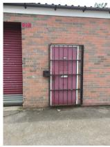
The doors to the rear of the building were fitted with fire escape hardware and a security drop bar system for when the unit is unoccupied.
