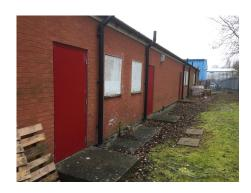
All doors were supplied with a powder coat finish. The existing doors were cleared from site by our engineers. All new door drames were mastic selaed by A&C.
