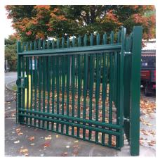
We upgraded the gate leaves and posts with more heavier duty steel box sections. The steel was powder coated including the palisade fencing to match to match the existing.
