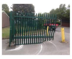
Due to the estate being exposed to further criminal activity. Our client required a replacement gate and fencing urgently. Our factory was able to fast track manufacture a new pair of gate leaves and posts. A&C engineers dug out the damaged gates and palisade fencing.
