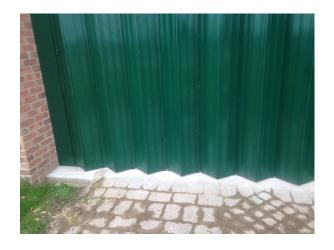
The Doors were supplied with a green powder coat finish. Galvanised pressed metals flashings powder coated to match the new doors were fixed to the door jambs. The flashings closed off the gaps between top of the walls and the door soffits.
