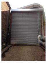
Our solution to the problem was to reduce the roller shutter curtain in width. Cutting the shutter laths and using the offcuts to form a side infill panel above the pipes. A plasma cut steel plate profile was also fitted around the pipes to seal all the gaps.
