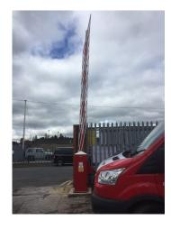
A&C engineers dismantled and removed the existing steel gates and installed a new pair of Traffic Barriers, each with a 4.5M span. To prevent access by pedestrians a double skirt was fitted to each barrier. Automatic operation for vehicles was by induction loops to both sides of the opening.
