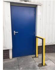
A&C was asked if we could provide a solution to the problem. Or solution was to manufacture and install two new powder caoted Door Restraint Frames.
