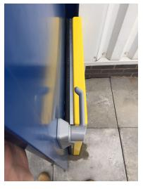
Each door leaf was fitted with aluminium carriers and rubber seals to the top and bottom of the frrame legs. The frames were cast into the ground exactly at the 90 degree opening point, preventing the overtravel and dampening the opening force of the door leaves.
