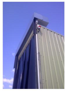
Each shutter was mounted on the outside of the unit, fully enclosed from the elements with a hood, fascia and motor cover. Supplied with wind anchored guides and a 400x4mm black PVC strip curtain to hide the opening from view when the shutter is open.
