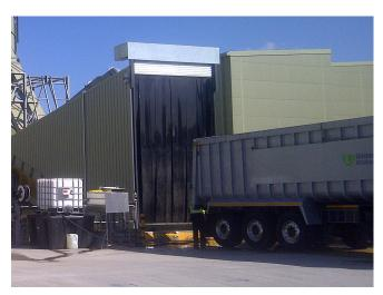
A&C Maintenance Ltd supplied & installed 2No. Safeguard 76 roller shutters to the incinerator sludge hoppers. The shutters were tall enough to allow the arctic lorries to tip the sludge into the hoppers.
