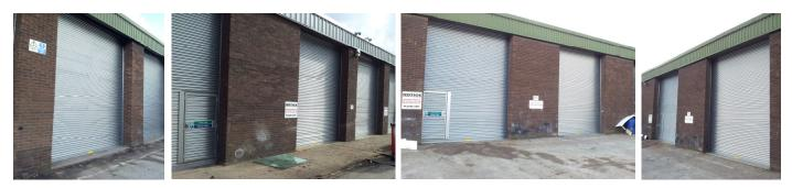
The contract involved the dismantle & removal from site of 21No. Bi-folding scissor action doors, supply & installation of 19No. Handchain Operated Roller Shutters 3500mm(W) x 5000mm(H) including independent safety brakes, 2No. Electrically Operated Roller Shutters 3500mm(W) x 5000mm(H).
