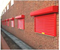
Our security shutters have a small compact shutter box as standard which includes mitred corners instead of rectangular. This proved to be successful in securing the project as our product was not industrial looking.
