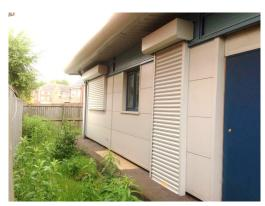
A&C Maintenance Ltd was able to overcome the facade problem by manufacturing bespoke endplates, guides & hood covers. With our own plasma cutting system we profile cut the endplates and guide angles to snugly fit around the facade profile. All the shutter parts we powder coated to match the facade colour & making the shutters blend in with the building.
