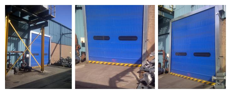
Activation of the doors are via induction loop sensors, inside & outside. Cutting of the loop slots and civil works were also carried out by A&C Maintenance Ltd.
