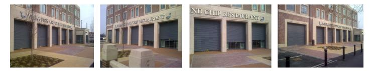
Specification included operation by single phase, 240 volt tube motors, lockable key switches and powder coat finish to shutter curtain, side guides and coil casing.
