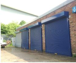
Due to the height being higher than a standard door opening a hook & pole was provided to help pull down each shutter. Locking is by means of a bullet lock & housing to each side guide with 2No. Keys per cylinder. All shutters were powder coat finished Blue RAL 5003.
