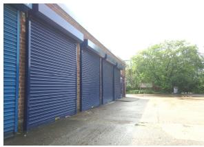
A&C Maintenance Ltd were awarded the contract for all of the roller shutters. Operation was by manual sprung balanced barrels, push up/pull down operation. Within the curtain were flush mounted lifting handle at chest height to help with opening & closing the shutters.
