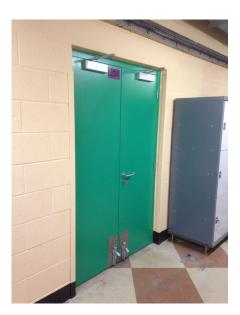
A&C Maintenance Ltd supplied & installed 2No. Double leaf steel 2 hour fire resistant doors with anti-jemmy astragal & frame studs. Hardware consisted of lock & lever handles, slimline door closer, leaf selector, flush bolts, floor bolt and floor mounted stops.
